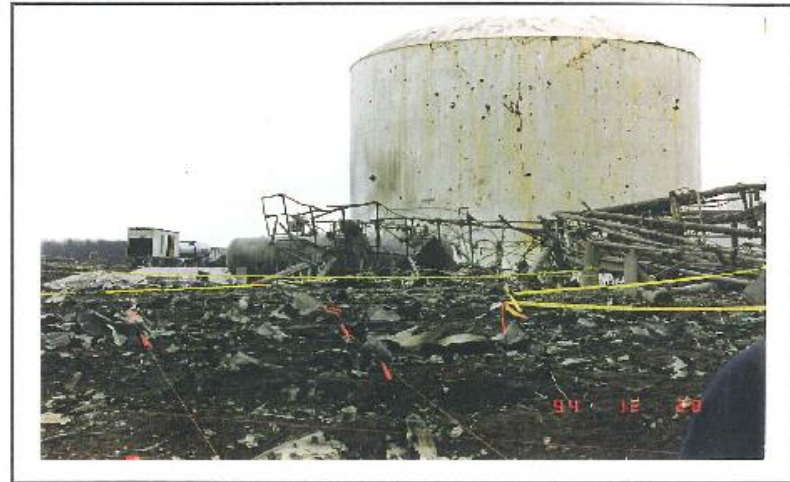
Photo 8 - 12 Water Tank Damage (Ammonia Tank Background)
